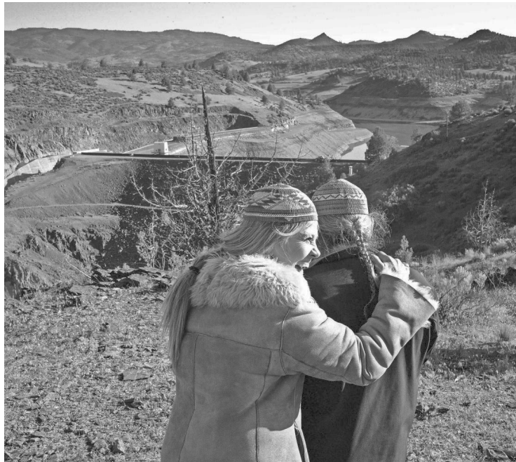
Karuk Tribal member Lisa Hillman, left, gives her husband, Leaf Hillman, a hug on an overlook above Iron Gate Dam as crews begin the removal of the top layer of the earthen dam that blocks the Klamath River east of Yreka, Calif., on May 1. CHRIS PIETSCH/THE REGISTER-GUARD
